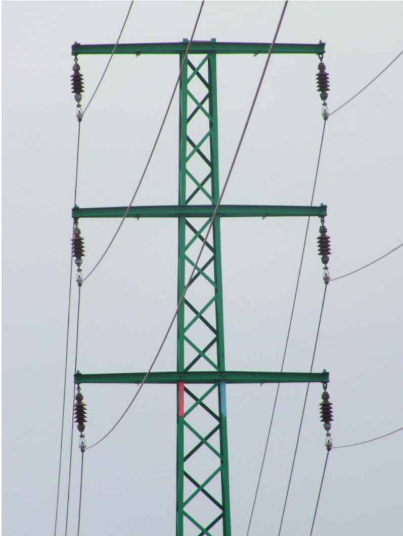
Figure B.8: Medium voltage pole with suspended insulators for double-circuit line. Source: Raptor Protection of Slovakia
