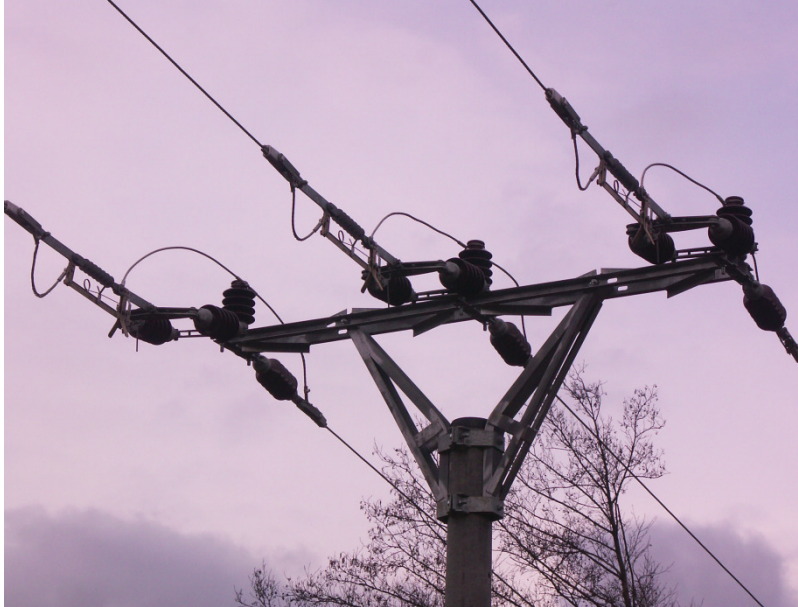
Figure 4.10: Strain poles with exposed jumper wires passing over the pin-insulators above the cross-arms are the most dangerous configuration responsible for many recorded electrocution fatalities. Source: Raptor Protection of Slovakia
