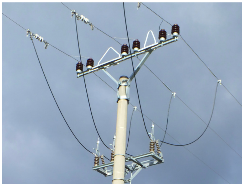
Figure C.6: Old types of switch disconnectors can be replaced with new one attached below the main cross-arm, as preferred in Slovakia. Source: Raptor Protection of Slovakia
