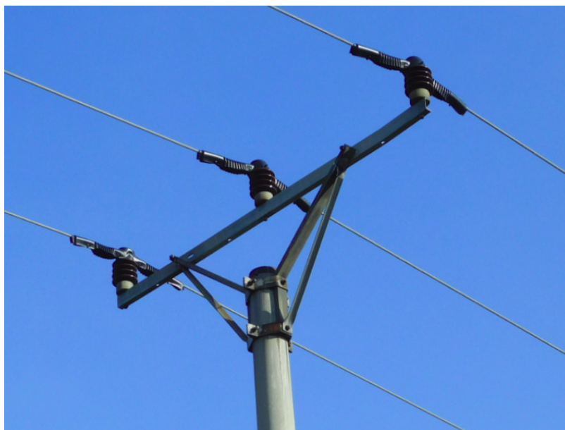
Figure C.3: Insulation caps for pin-type pylons in Czech Republic. Source: AOPK ČR
