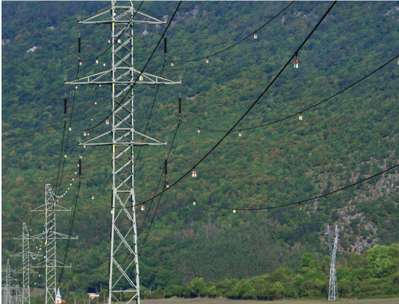
Figure D.5: For high voltage lines up to 110 kV is important to increase the visibility of all phase conductors and the earth (shield) wire on the top. Source: Raptor Protection of Slovakia
