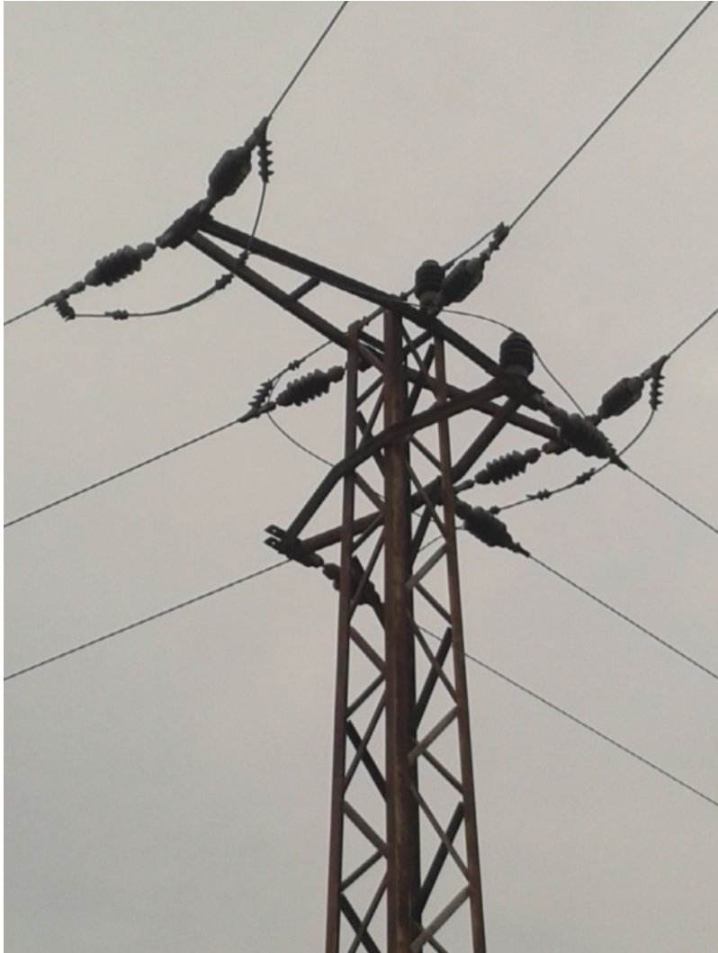
Figure B.4: Branch pole of 22 kV line in Czech Republic. Construction is very similar to poles used in Slovakia. Source: AOPK ČR
