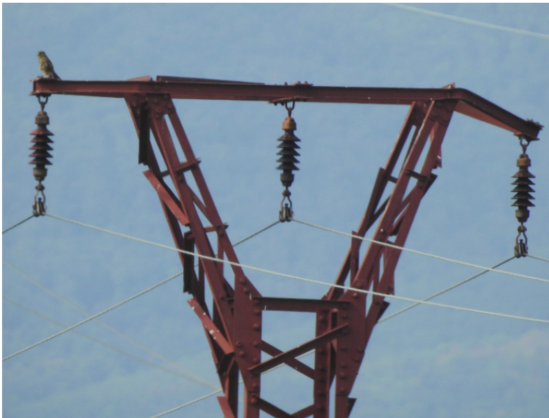
Figure B.7: Medium voltage pole with suspended insulators for single-circuit line. Source: Raptor Protection of Slovakia
