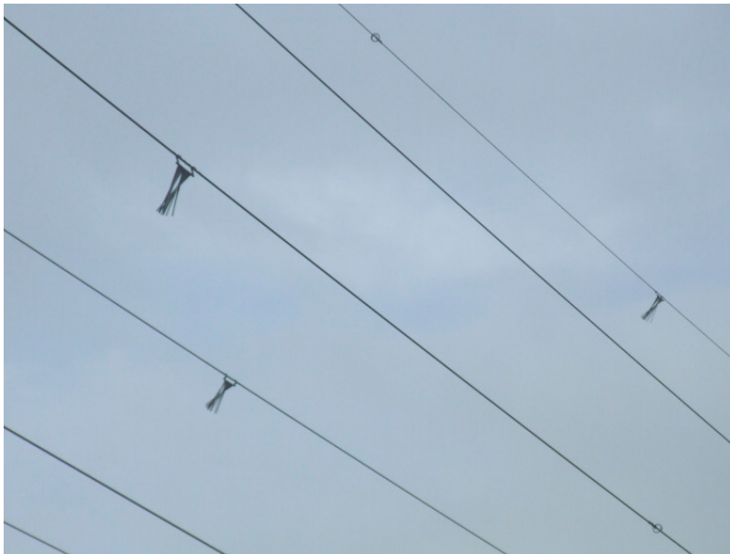
Figure D.8: Different combination of bird diverters (spiral and devices with movement parts) can be used to increase the visibility of line. Source: Raptor Protection of Slovakia
