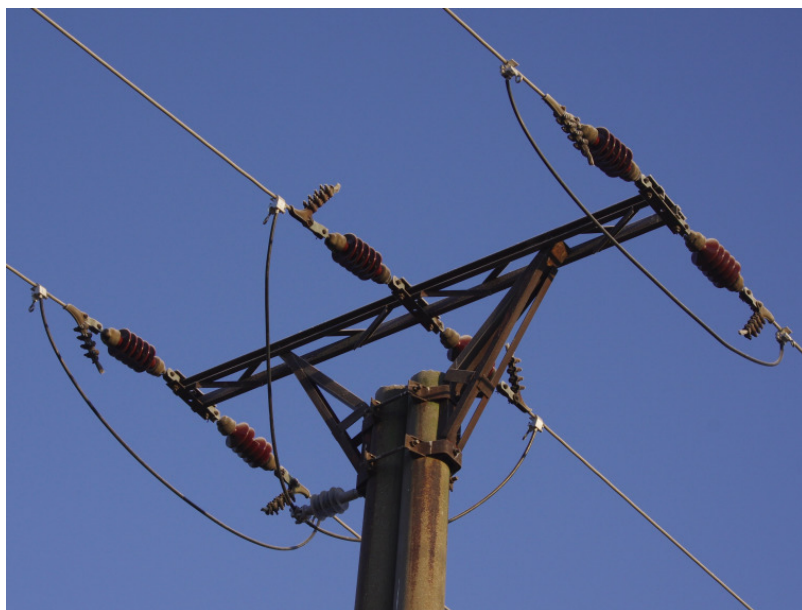
Figure C.5: Effective solutions for bird protection in Slovakia. Dangerous jumper wires were placed under the cross-arm with fully insulated phase conductors. Source: Raptor Protection of Slovakia
