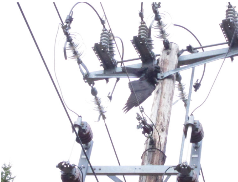
Figure B.5: Unisolated jumper wires on 10 kV pole in Sweden. Source: EON Sweden
