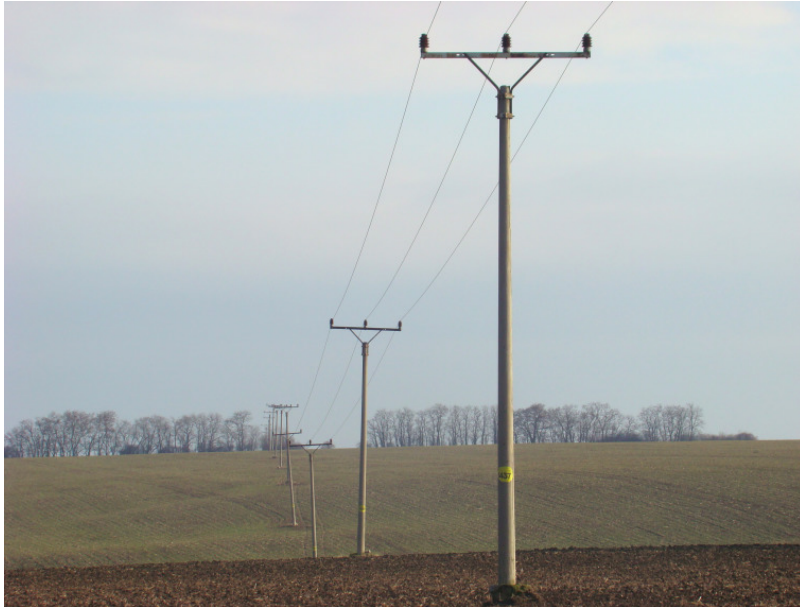
Figure A.3: Medium voltage pole of 22 kV distribution line in Slovakia. Source: Raptor Protection of Slovakia
