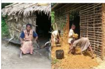
Construction of new and improved houses by the indigenous people
